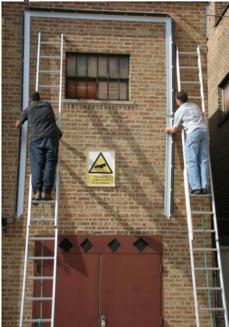
Mounting frame sides to our building.
